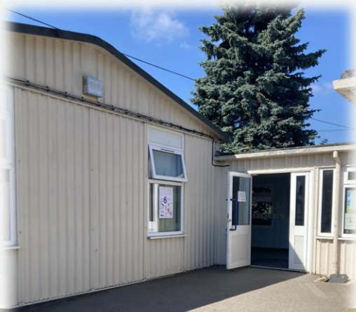
Year 5 Entrance and Exit Door 14
